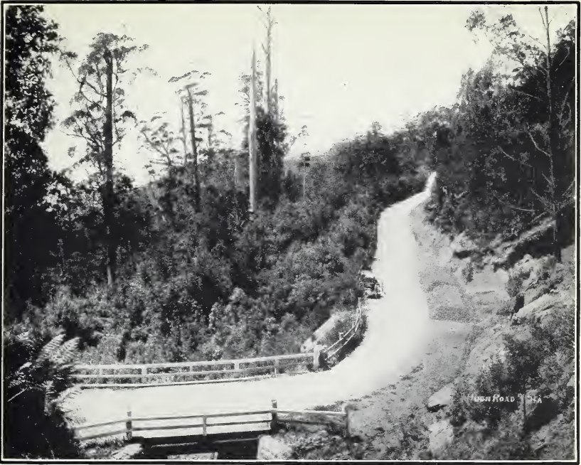
FIG. 1.—ROAD IN TASMANIA, SHOWING STACKS OF STONE FOR REPAIRS.
